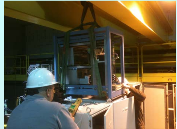
New SMPC electronics rack installation
