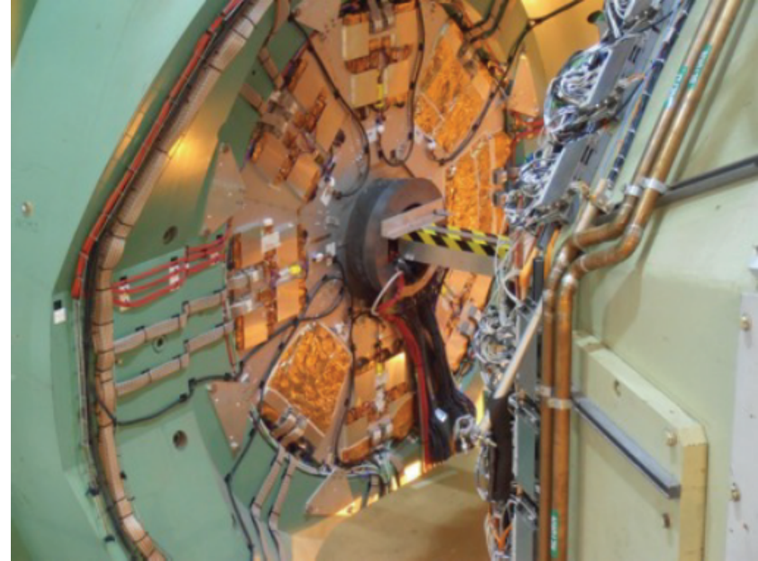
North RPC Station 1
